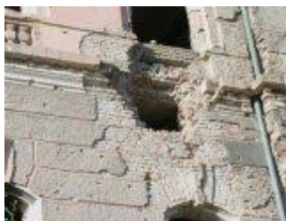
155mm HE round, 10 inch thick brick wall
